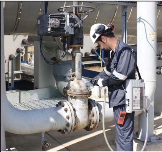
Leak Detection and Repair Program
